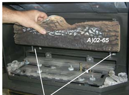
Pins on Rear Log Support
